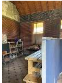
Rock Island Train Station (Shorter College Business Hub Site)
