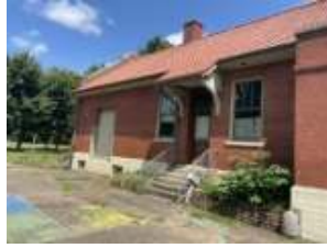
Rock Island Train Station (Shorter College Business Hub Site)
